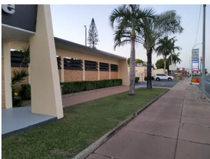
Photo uploaded: Building 1 Environmental 20 Oct 2023 7:13pm
