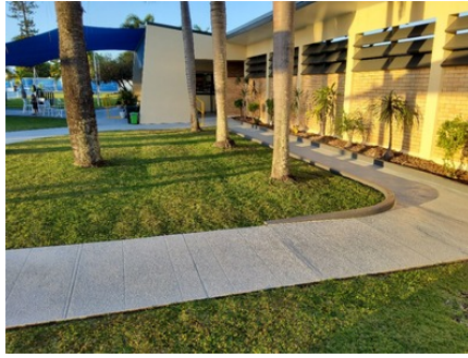
Photo uploaded: Building 1 Formal pathway surrounding building 20 Oct 2023 6:38pm
