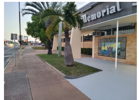
Photo uploaded: Building 1 Environmental 20 Oct 2023 7:13pm
