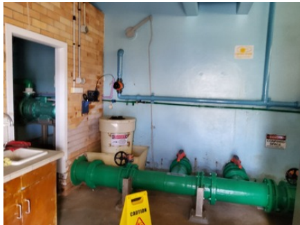
Photo uploaded: Building 2 Ceiling height - lowest point 18 Dec 2023 12:37pm
