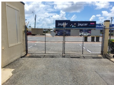
Photo uploaded: Supporting Amenities 1 Truck access 18 Dec 2023 11:55am
