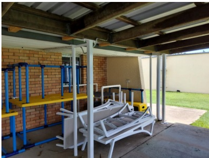
Photo uploaded: Building 3 Ceiling height - lowest point 18 Dec 2023 12:50pm
