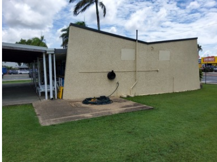
Photo uploaded: Building 3 Overall condition of building exterior 18 Dec 2023 12:59pm
