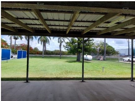
Photo uploaded: Building 3 Ceiling height at highest point 18 Dec 2023 12:51pm
