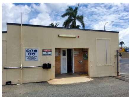
Photo uploaded: Building 2 Utilities/plant room 18 Dec 2023 12:43pm
