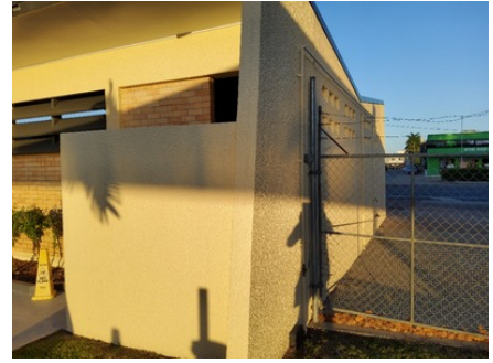
Photo uploaded: Building 1 Overall condition of building exterior 20 Oct 2023 6:38pm
