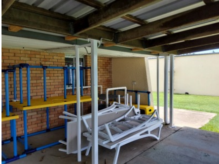
Photo uploaded: Building 3 Internal club/user storage area 18 Dec 2023 1:01pm
