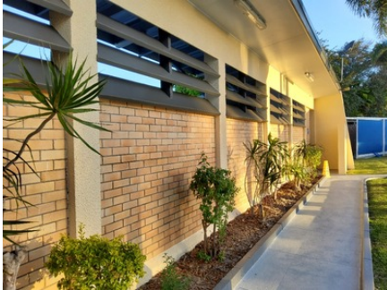
Photo uploaded: Building 1 Main external building materials 20 Oct 2023 6:37pm
