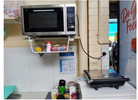
Photo uploaded: Building 1 Power outlets 18 Dec 2023 12:27pm
