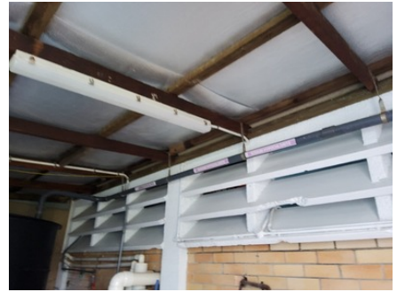
Photo uploaded: Building 2 Ceiling height at highest point 18 Dec 2023 12:38pm
