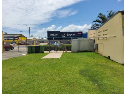
Photo uploaded: Building 1 External bin storage area 18 Dec 2023 12:04pm
