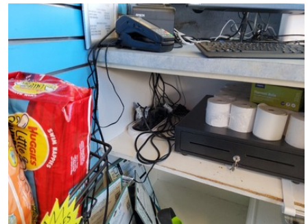
Photo uploaded: Building 1 Power outlets 18 Dec 2023 12:25pm
