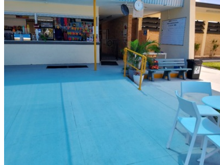
Photo uploaded: Building 1 Formal pathway surrounding building 18 Dec 2023 12:01pm
