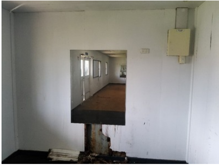
Photo uploaded: Building 3 Site issues - building 18 Dec 2023 1:11pm
