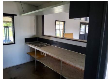
Photo uploaded: Building 3 Internal kitchen/kiosk servery 18 Dec 2023 1:06pm
