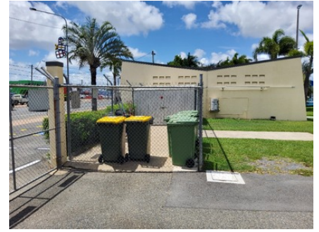
Photo uploaded: Building 1 External bin storage area 18 Dec 2023 12:03pm
