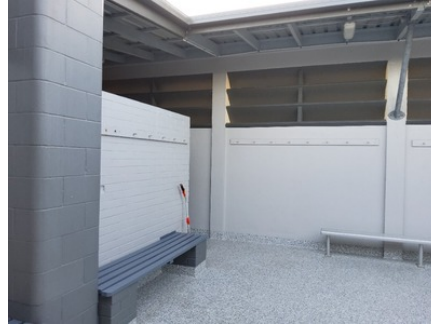
Photo uploaded: Building 1 Ceiling height at highest point 20 Oct 2023 6:36pm
