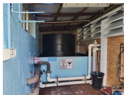
Photo uploaded: Building 2 Power outlets 18 Dec 2023 12:44pm
