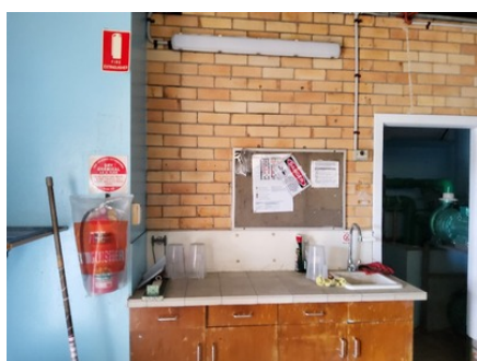
Photo uploaded: Building 2 Utilities/plant room
