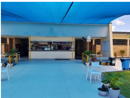
Photo uploaded: Building 1 Administration 18 Dec 2023 12:17pm
