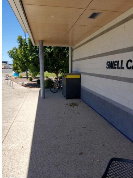
Photo uploaded: Building 1 External bin storage area 11 Oct 2023 2:10pm
