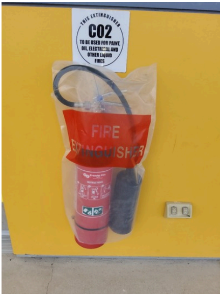
Photo uploaded: Building 2 Main external building materials 12 Oct 2023 12:14pm Render
