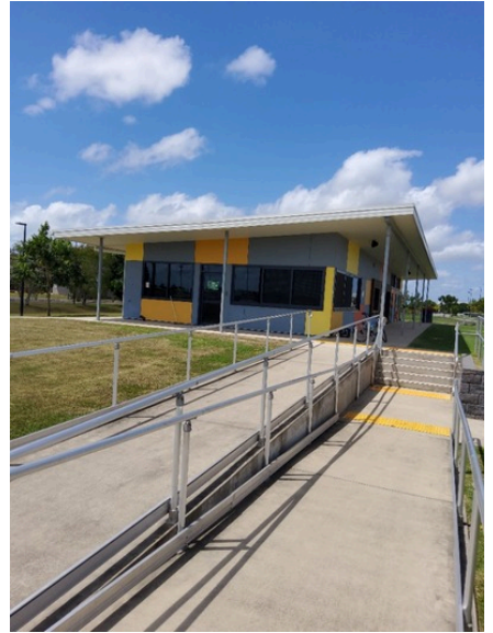
Photo uploaded: Building 2 Building access 12 Oct 2023 12:12pm
