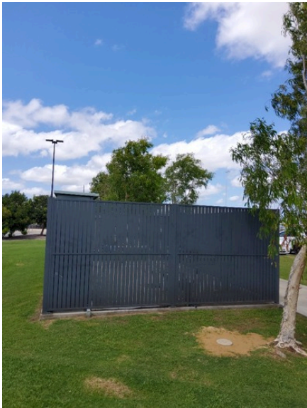
Photo uploaded: Building 2 Misc 12 Oct 2023 2:08pm Unsafe facilities purpose.
