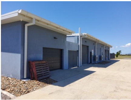
Photo uploaded: Building 1 External bin storage area 11 Oct 2023 3:08pm
