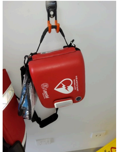
Photo uploaded: Building 2 Defibrillator machine 12 Oct 2023 12:31pm
