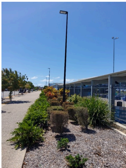
Photo uploaded: Supporting Amenities 1 Accessible pathways 11 Oct 2023 12:26pm
