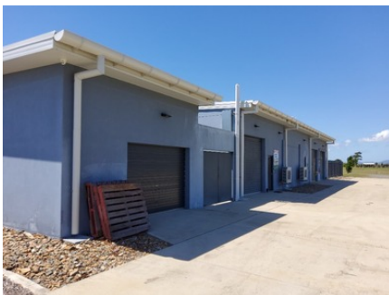
Photo uploaded: Building 2 External bin storage area 12 Oct 2023 12:23pm
