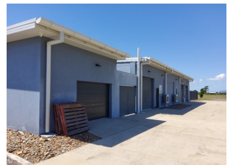
Photo uploaded: Building 1 Utilities/plant room 11 Oct 2023 2:19pm
