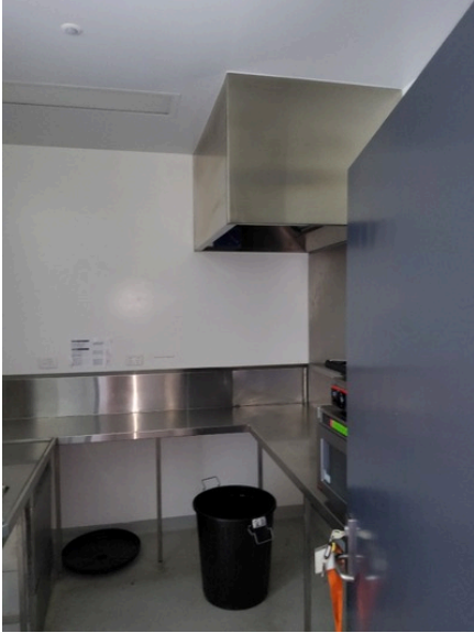
Photo uploaded: Building 2 Canteen/kitchen 12 Oct 2023 12:41pm
