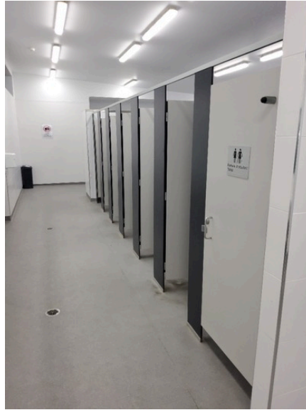
Photo uploaded: Building 1 Building toilets 11 Oct 2023 3:16pm
