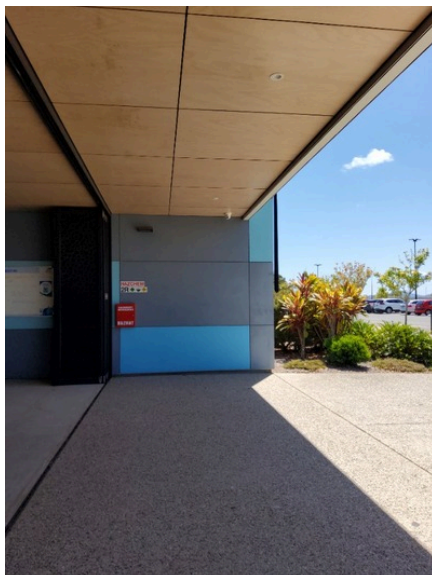
Photo uploaded: Building 1 Ceiling height - lowest point 11 Oct 2023 2:02pm
