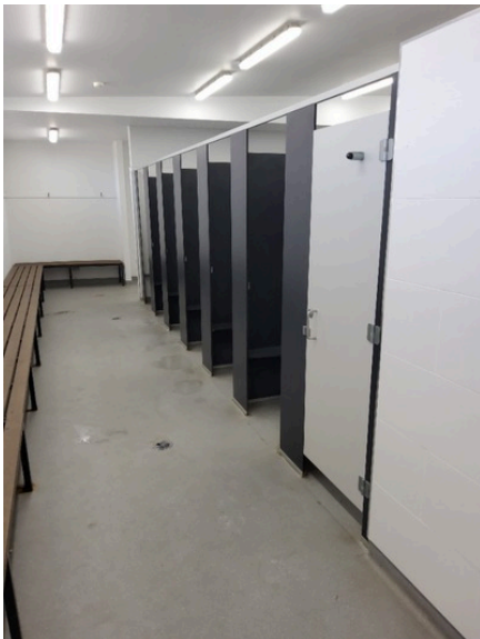
Photo uploaded: Building 1 Building toilets 11 Oct 2023 3:17pm
