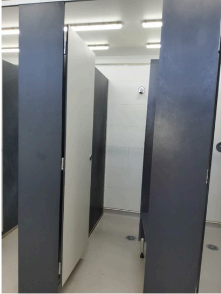
Photo uploaded: Supporting Amenities 1 Spectator toilets 11 Oct 2023 1:44pm
