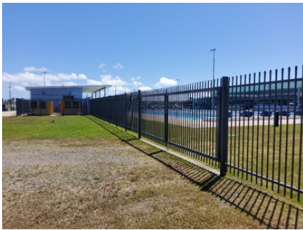
Photo uploaded: Supporting Amenities 1 Gated access points 11 Oct 2023 1:50pm
