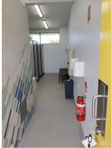
Photo uploaded: Building 2 Building toilets 12 Oct 2023 2:03pm Male toilet.
