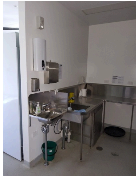
Photo uploaded: Building 2 Canteen/kitchen 12 Oct 2023 12:42pm
