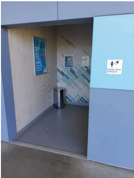
Photo uploaded: Building 1 Building toilets 11 Oct 2023 3:15pm
