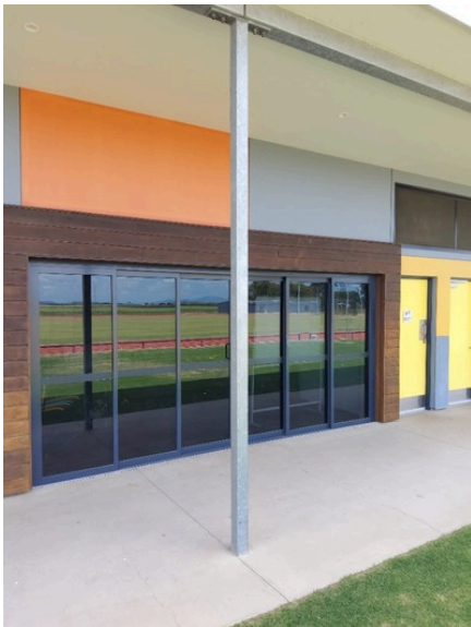
Photo uploaded: Building 2 Building access 12 Oct 2023 11:05am
