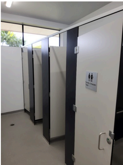
Photo uploaded: Building 2 Building toilets 12 Oct 2023 2:04pm Female toilet.
