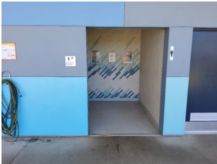
Photo uploaded: Supporting Amenities 1 Spectator toilets 11 Oct 2023 1:47pm
