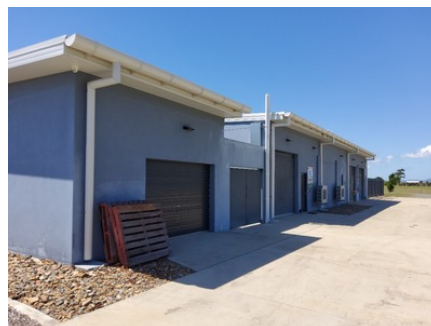
Photo uploaded: Building 1 External goal or equipment storage 11 Oct 2023 3:09pm
