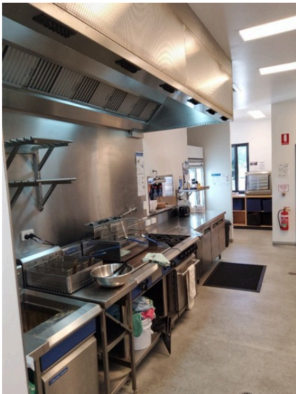
Photo uploaded: Building 1 Canteen/kitchen 11 Oct 2023 2:24pm
