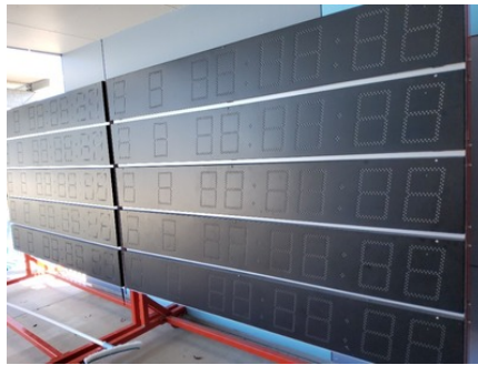
Photo uploaded: Building 1 Overall condition of building exterior 11 Oct 2023 3:07pm
